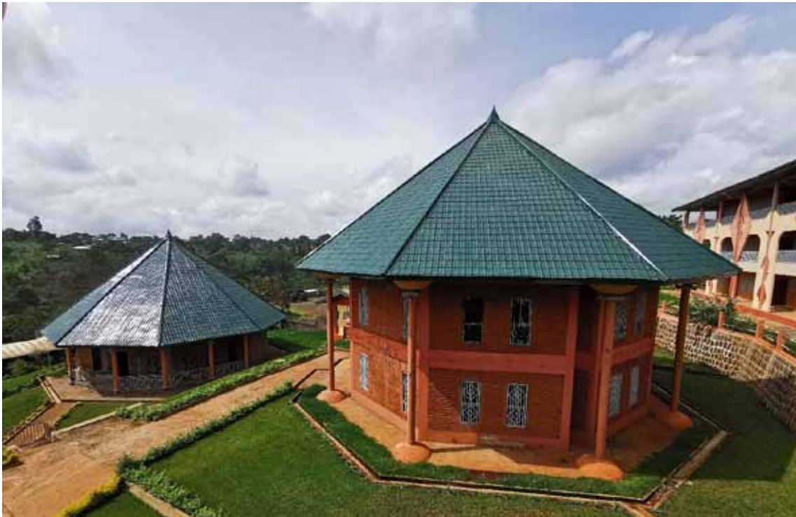
Fig. 106_ Multimedia building and canteen with new roofing after the fire
