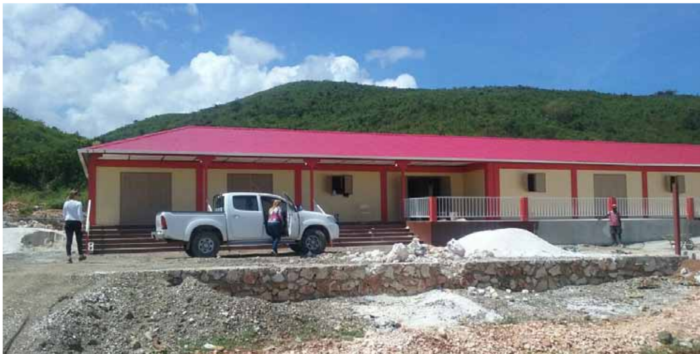
Fig. 108_ New construction of evacuation centre in Miragoâne
