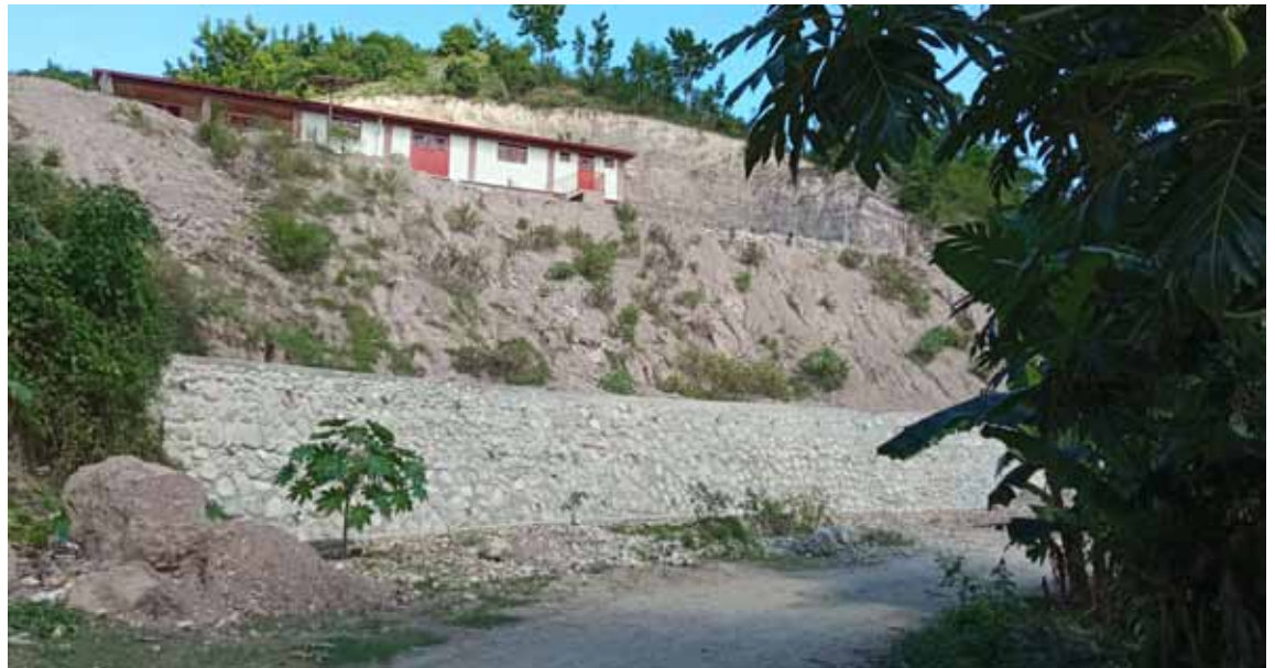
Fig. 111_ View from the valley to the evacuation centre and the lower retaining wall in Baradères
