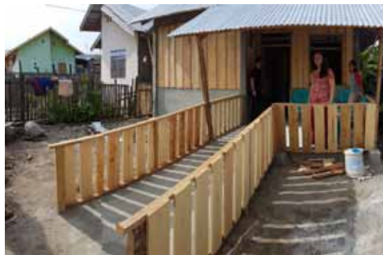
Fig. 66_ Example of ramp in Indonesia (left picture)
