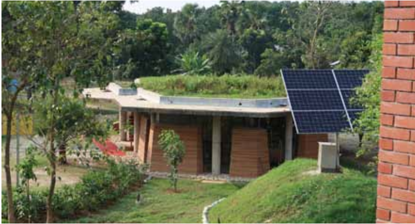
Fig. 55_ Green roof with intensive greening in Bangladesh
