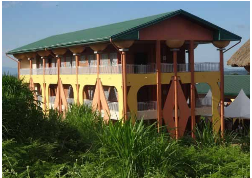
Fig. 101_ New administration building (3-storey)
