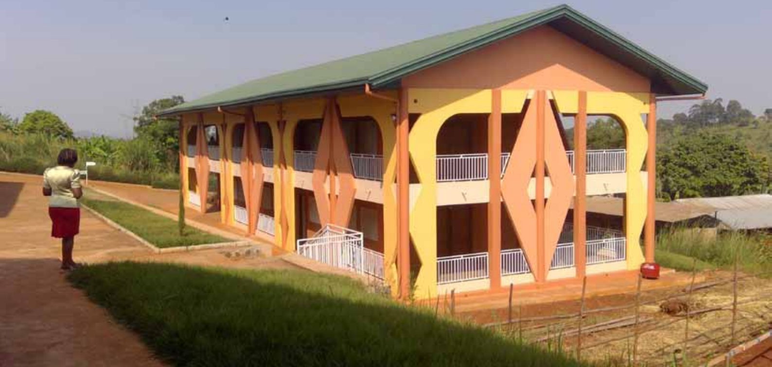
Fig. 100_ New administration building (2-storey)
