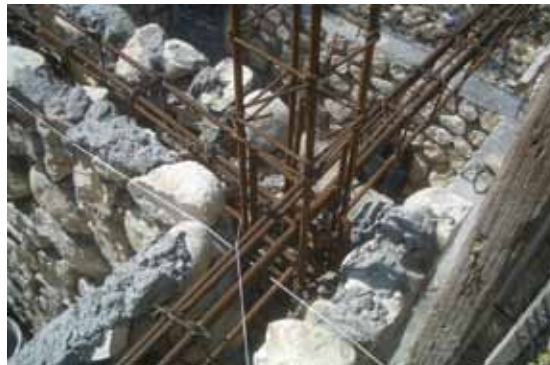
Fig. 24_ Example of confined masonry (left picture)
