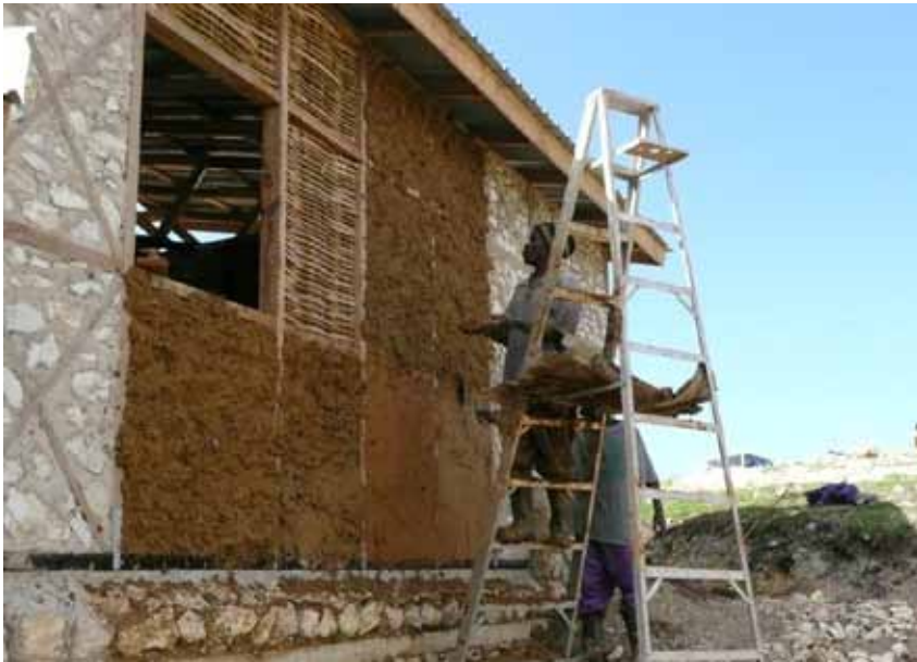
Fig. 81_ Construction site of model house
