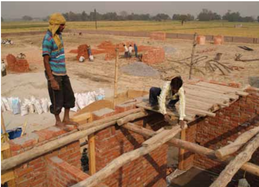
Fig. 92_ Formwork of the concrete work
