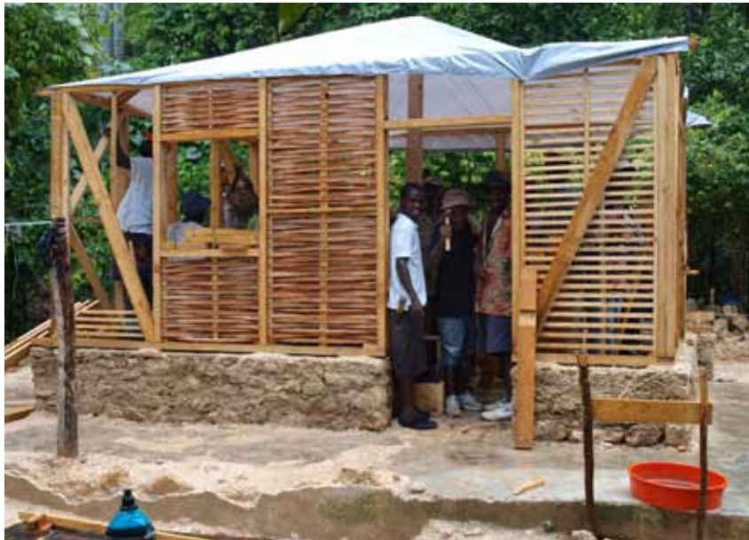
Fig. 83_ One of the first houses used for trainings and demonstration (Clissage-technic)
