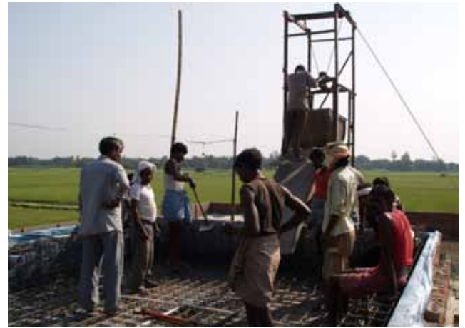
Fig. 93_ Concrete works: prefabrication of lintels; self-made spacers to ensure the concrete cover ; concrete work with lift of the ceiling
