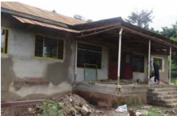
Fig. 130_ Building after modernization with accessible parking space (right picture)
