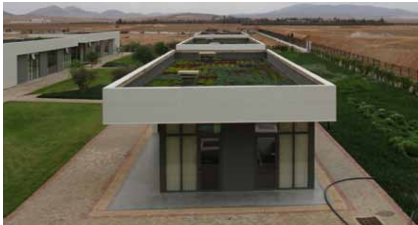
Fig. 56_ Green roof with extensive greening in Morocco
