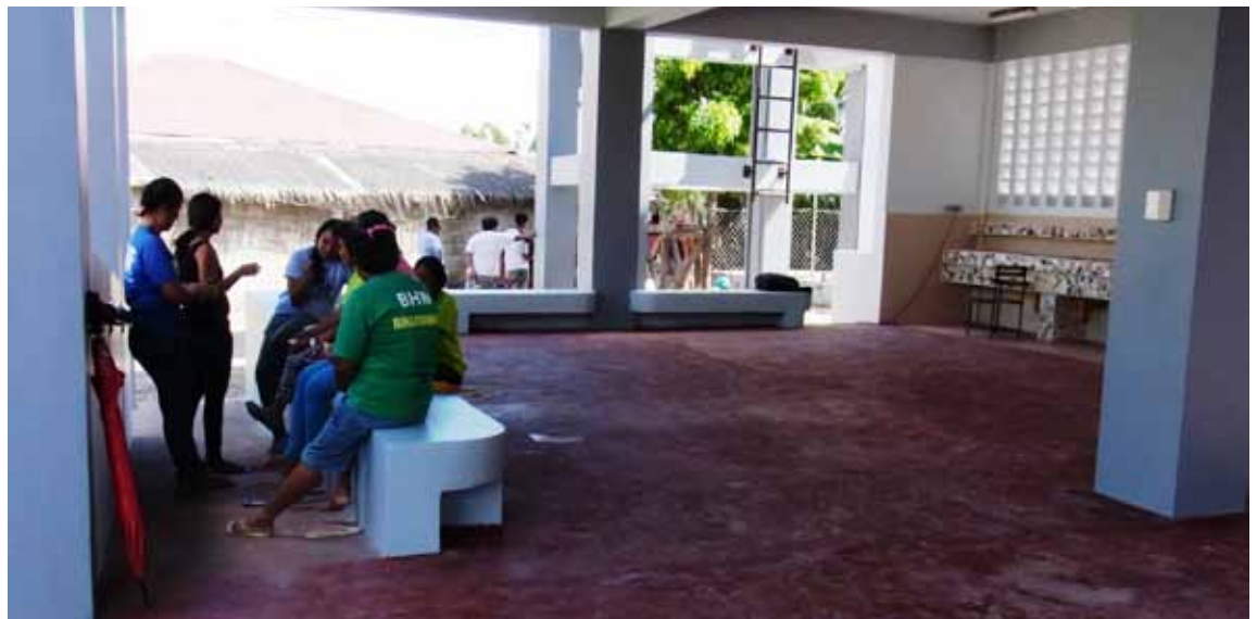
Fig. 137_ View on ground floor area with ramp & kitchen
