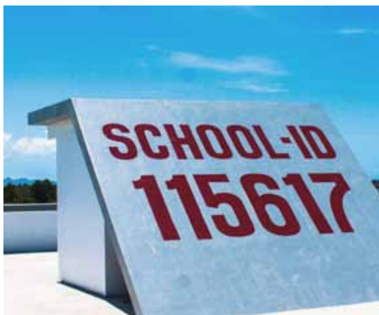
Fig. 141_ School ID on the roof
