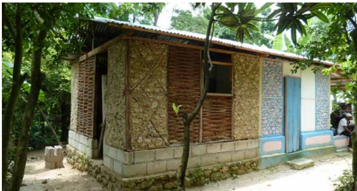
Fig. 85_ Rivière Froide: Base modul with extension by beneficiaries, clissage combined with stone infill
