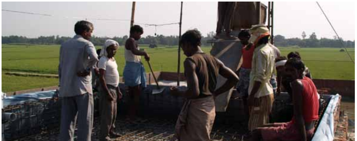
Fig. 4_ School construction in India
