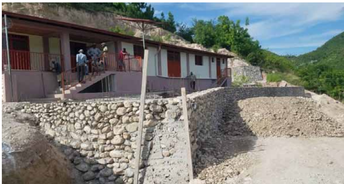
Fig. 112_ Evacuation centre with upper retaining wall in Baradères
