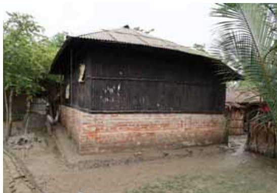
Fig. 32_ Example of building elevated on plinth to avoid floods
