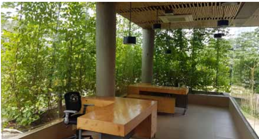
Fig. 57_ Green facade in Bangladesh
