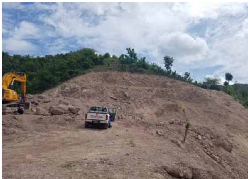
Fig. 110_ Site prepara- tion before const- ruction in Baradères
